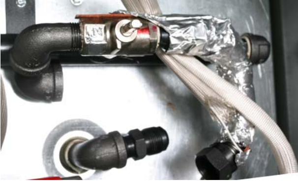
Figure 3: The front flush hose is shown disconnected.
