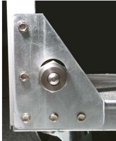
Figure 6: The new rear-discharge plumbing is shown extending through an existing cabinet gusset. The quick-disconnect is in place.
