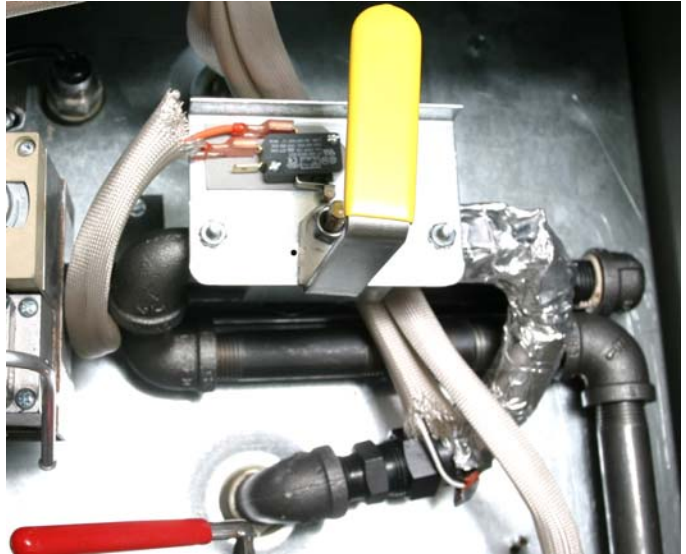
Figure 4: The plumbing for the rear discharge system is shown in place. The valve bracket, with the stop pin removed, allows 180° rotation of the handle, allowing for a return and discharge position.
